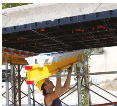
⑥ REMOVAL OF THE H BEAM
