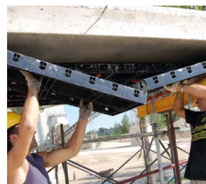
⑧ REMOVAL OF GEOPANEL
