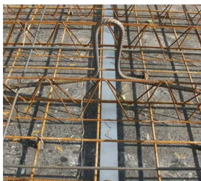
④ ADD THE REINFORCEMENT
