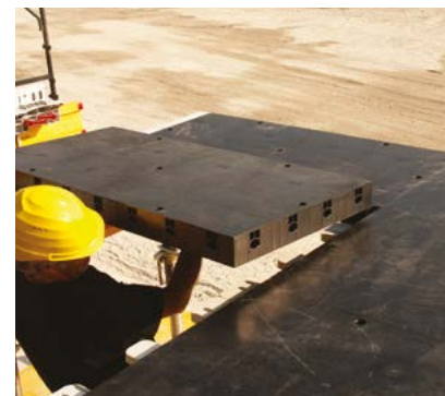
③ PLACE GEOPANEL
