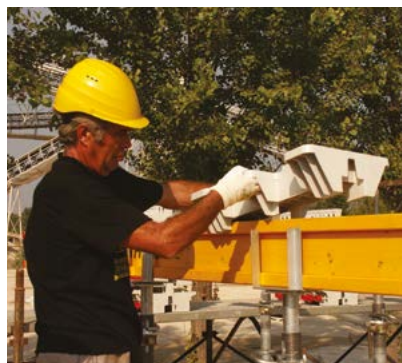
② PLACE THE H BEAMS
