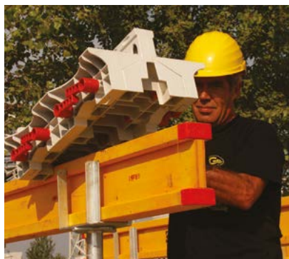
① PLACE THE Y BEAMS +WEDGE
