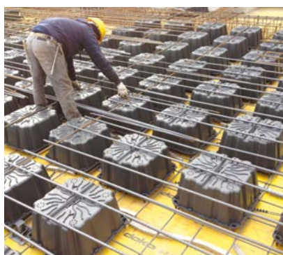
④ UPPER REINFORCEMENT INSTALLATION
