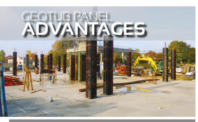
The light, reusable and modular system for the construction of square and rectangular columns
