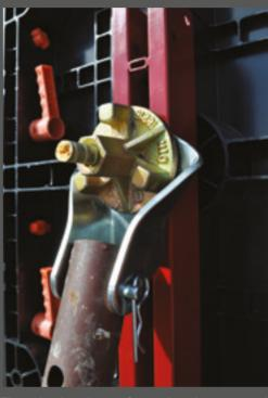
The shoring is performed using a steel bracket to connect push-pull props to the formwork. The brackets are available in various sizes to suit any commercially available props.
