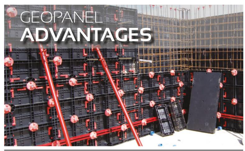
The only light, reusable and modular system for concrete wall production
