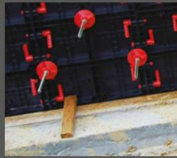
Anchoring to the ground to stabilise the formwork is simply done using timber.
