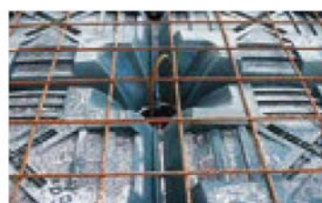
Reinforcement of the pillar with steel forks
