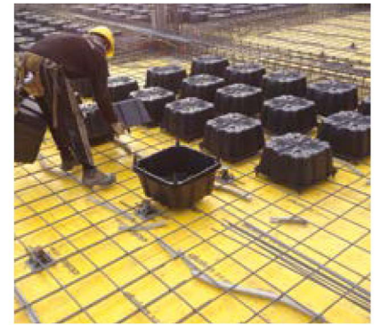
③ INSTALLATION OF NEW NAUTILUS
