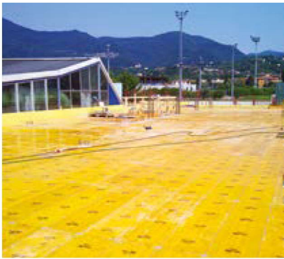
① BASE DECK PREPARATION
