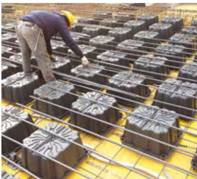
④ UPPER REINFORCEMENT INSTALLATION
